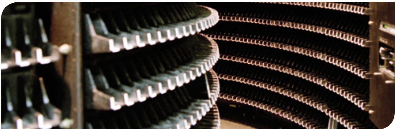
Lufthansa Systems: The latest technology helps reduce the energy consumption of data centers.
