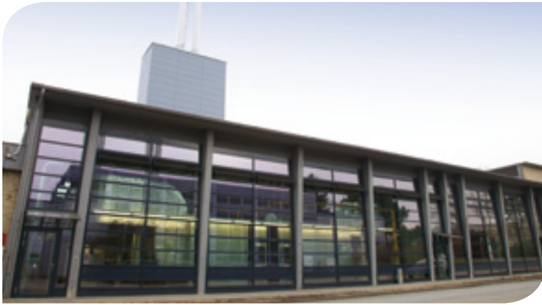
The new cogeneration plant of Lufthansa Technik AG in Hamburg.
