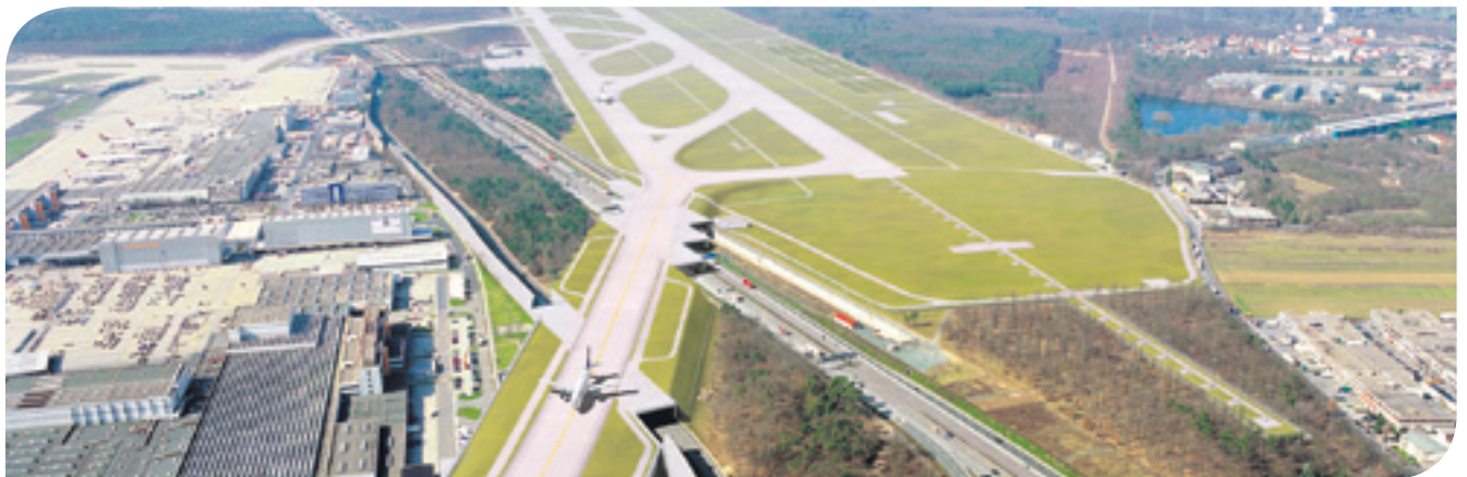
Frankfurt Airport's new Runway Northwest.
