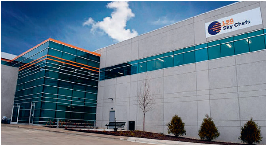
View of the state-of-the-art LSG Sky Chefs operation in Chicago, which was opened at the end of 2015. Constructed in accordance with LEED standards (Leadership in Energy & Environmental Design), this airline catering building is the first worldwide to have received the quality seal of the U.S. Green Building Council (USGBC).
